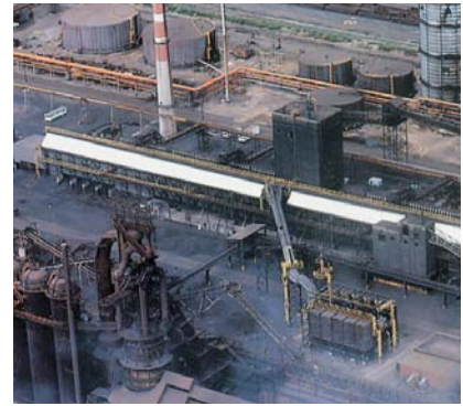
Dust collection system installed at a major steel manufacturing facility
